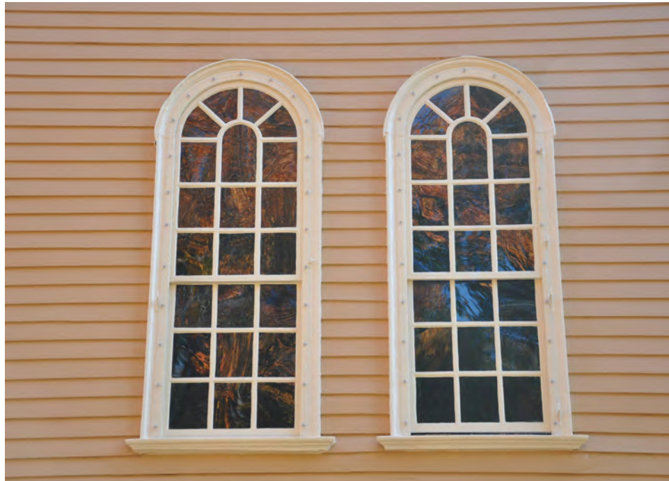
Figure 22. Old Ship Meeting House. West elevation – 1755 sash restored with new protective covers installed.
