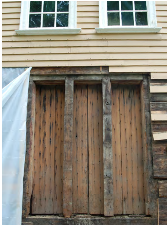
Figure 24. Old Ship Meeting House. Original 1681 doors uncovered in west wall; covered over in 1755.
