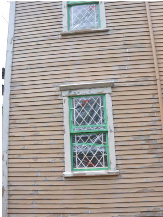
Figure 14. Old Ship Meeting House. Exterior painting – Surface preparation.
