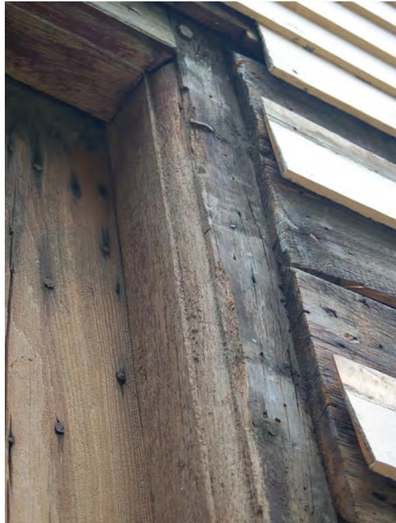
Figure 25. Old Ship Meeting House. Molding detail on casing of 1681 doors.
