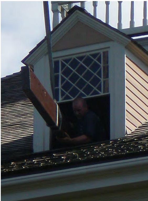
Figure 29. Old Ship Meeting House. Structural steel being guided into the attic through the south roof dormer window.
