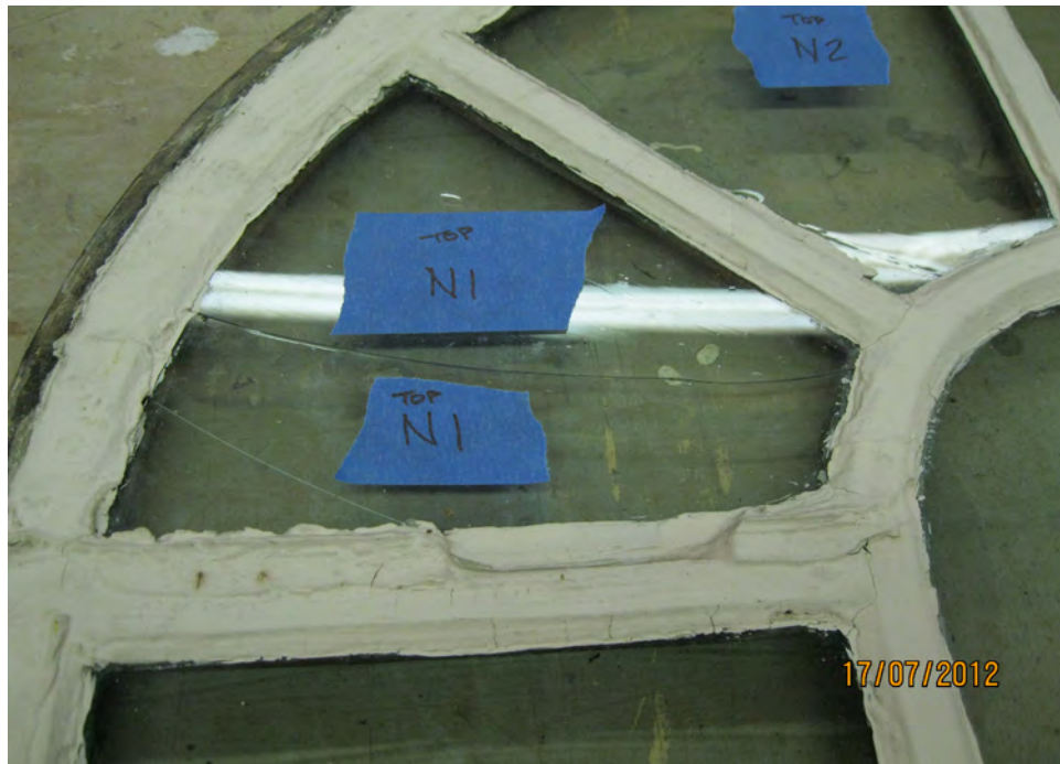
Figure 18. Old Ship Meeting House. 1755 sash – Detail of deteriorated glazing. Photo courtesy of David Webb.
