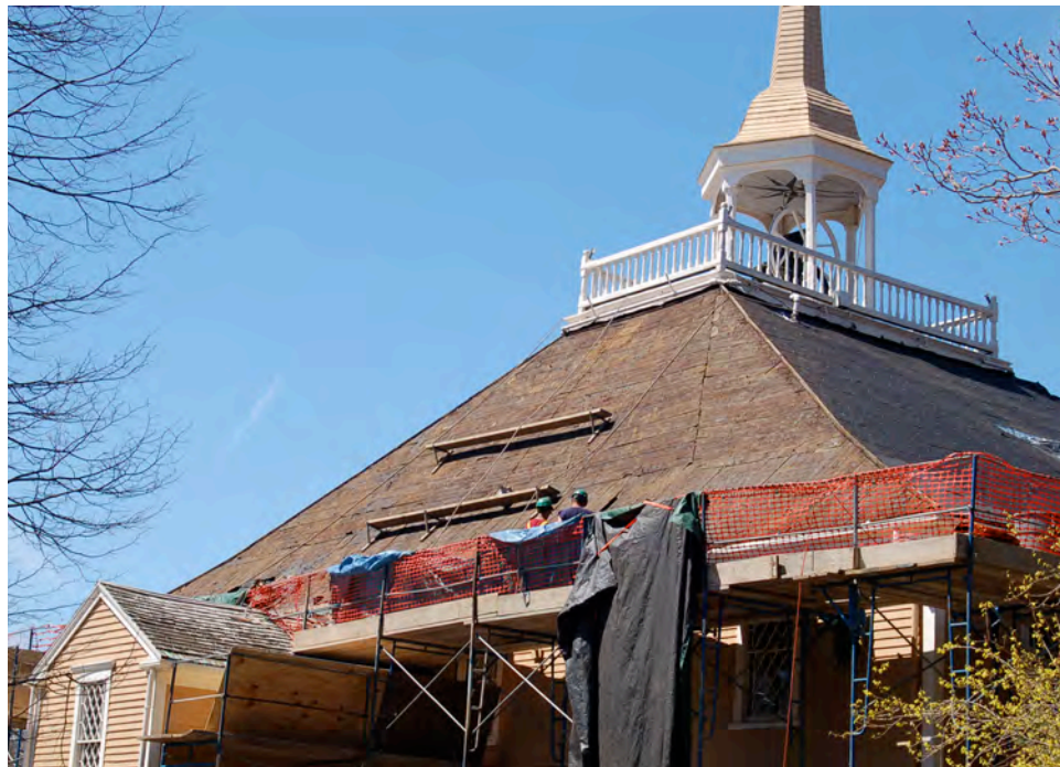
Figure 2. Old Ship Meeting House. East elevation – Wood shingle roof stripped, exposing historic sheathing boards.
