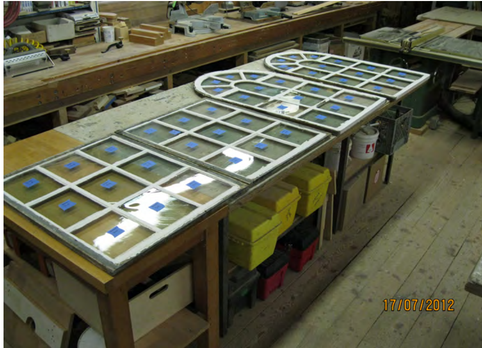
Figure 17. Old Ship Meeting House. 1755 sash removed for restoration. Photo courtesy of David Webb.
