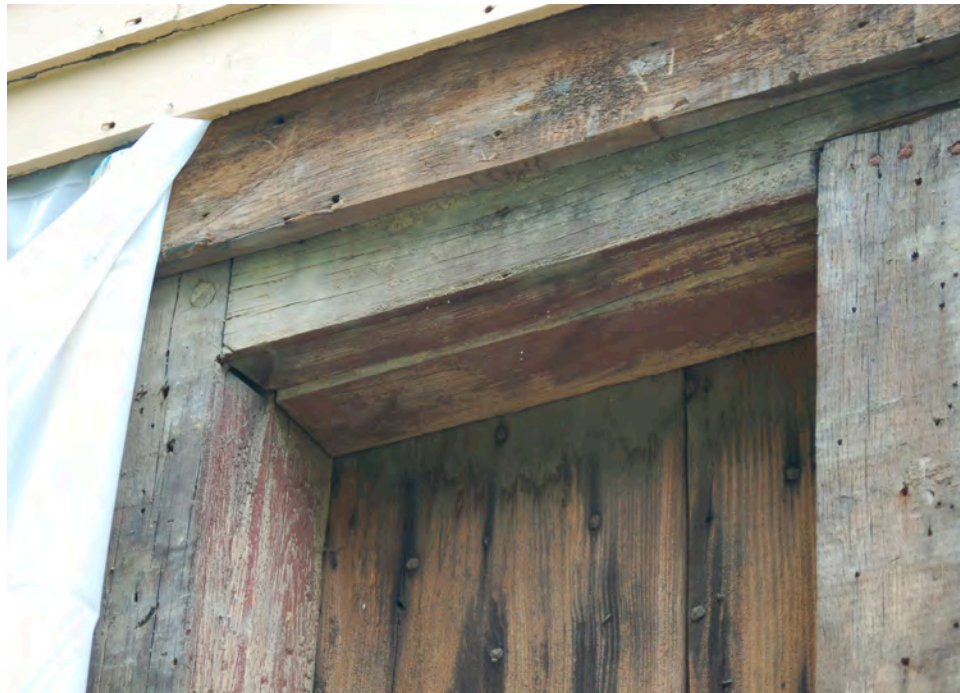
Figure 26. Old Ship Meeting House. Detail of red paint on casing of 1681 doors.
