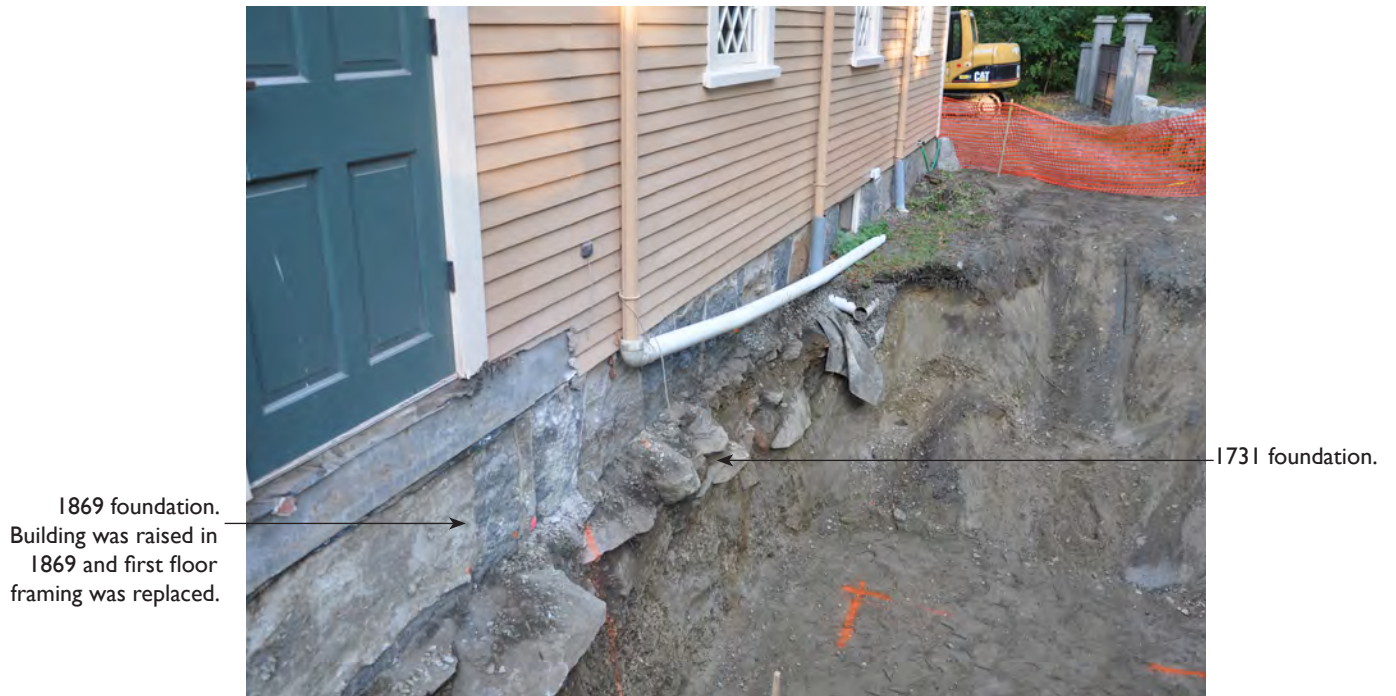
Figure 45. Old Ship Meeting House. North elevation – Privy excavation.
