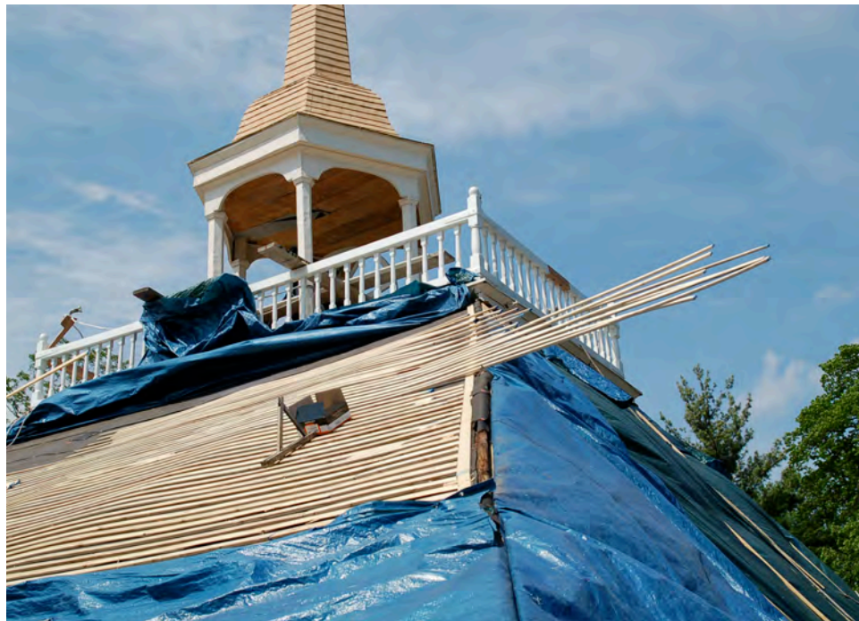
Figure 6. Old Ship Meeting House. South elevation – Installation of roof strapping.
