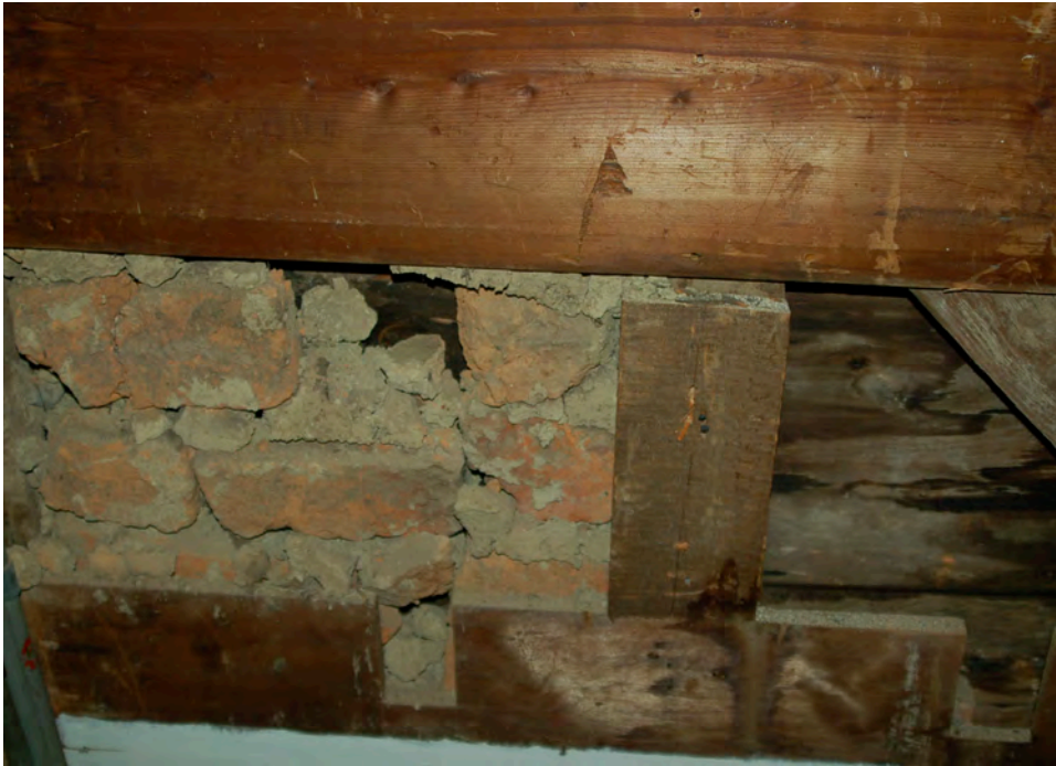
Figure 39. Old Ship Meeting House. East gallery wall showing 1681 brick and clay mortar nogging.
