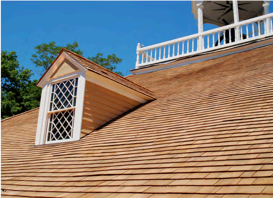
Figure 7. Old Ship Meeting House. South elevation – Restored dormer and wood shingle roof.
