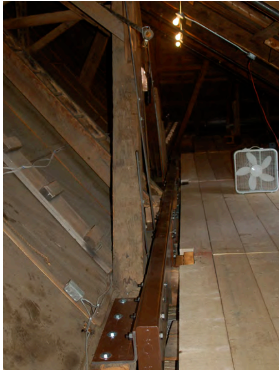
Figure 31. Old Ship Meeting House. New structural steel installed on north side of attic. Steel supplements the deflected plates of the original 1681 timber frame.
