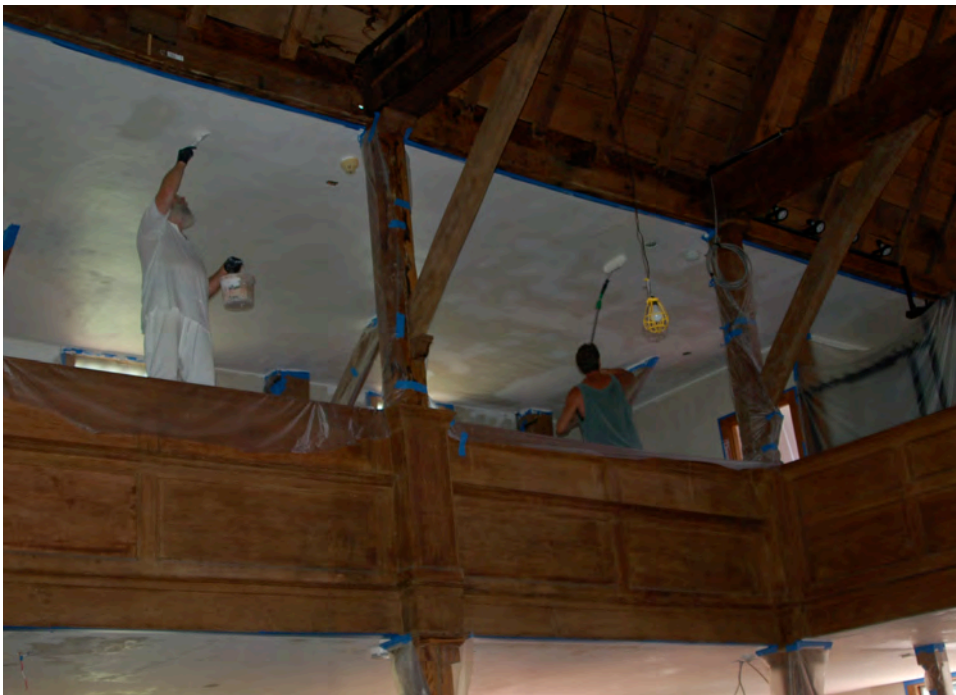
Figure 36. Old Ship Meeting House. Whitewash being applied to plaster walls and ceiling.
