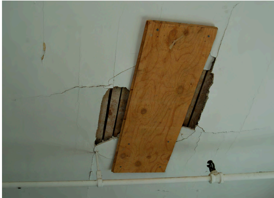
Figure 33. Old Ship Meeting House. Plaster failure requiring re-adhesion and patching.
