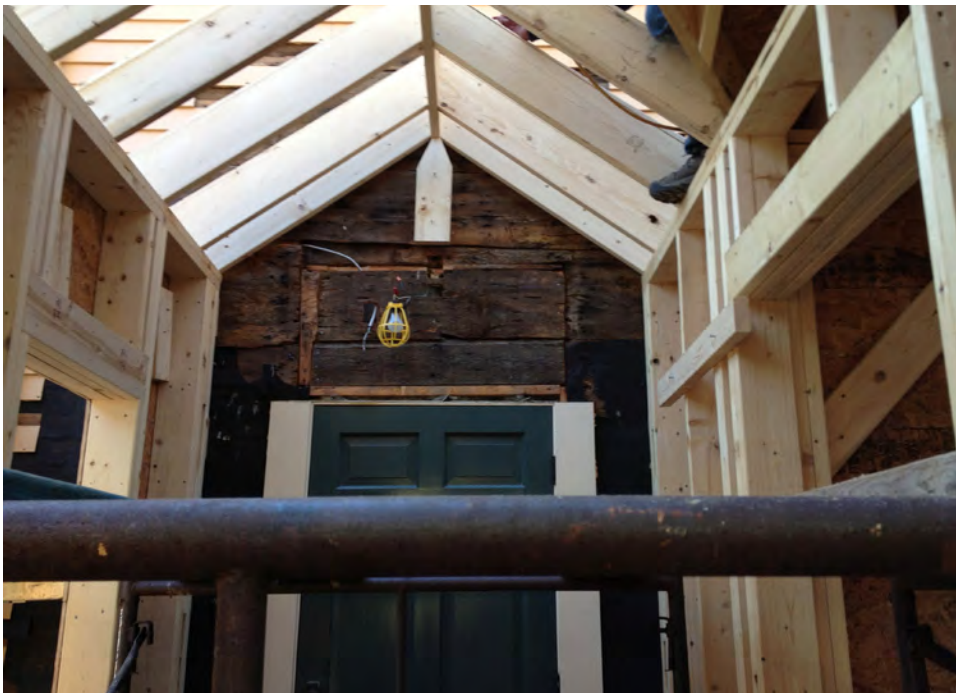
Figure 48. Old Ship Meeting House. Interior of privy during construction, showing window that was modified in the 1990's to create the door to the accessibility ramp.
