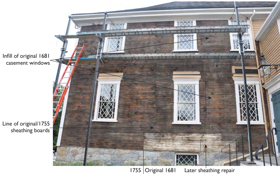
Figure 9. Old Ship Meeting House. Exterior carpentry repairs – East elevation – Modern clapboards removed and replaced. Note documentation of building history shown in sheathing boards.
