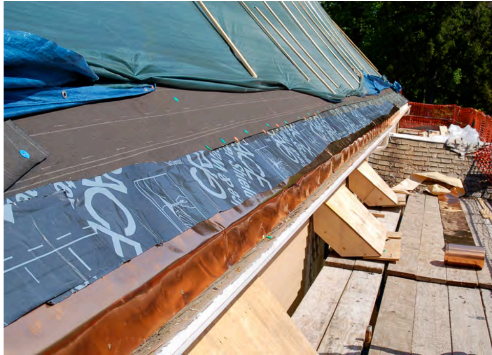
Figure 5. Old Ship Meeting House. East elevation – Installation of new ice and water shield at eave.
