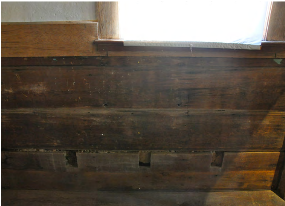
Figure 40. Old Ship Meeting House. East gallery – 1681 wall paneling showing pockets for original east gallery framing.
