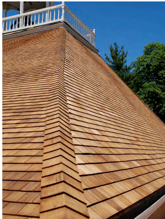
Figure 8. Old Ship Meeting House. Southeast corner of wood shingle roof showing woven hip.
