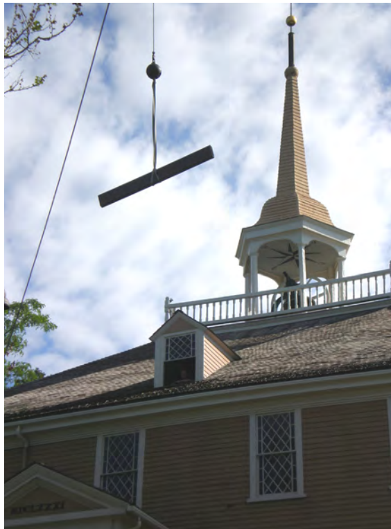
Figure 28. Old Ship Meeting House. Structural steel being lifted by crane into Meeting House attic.
