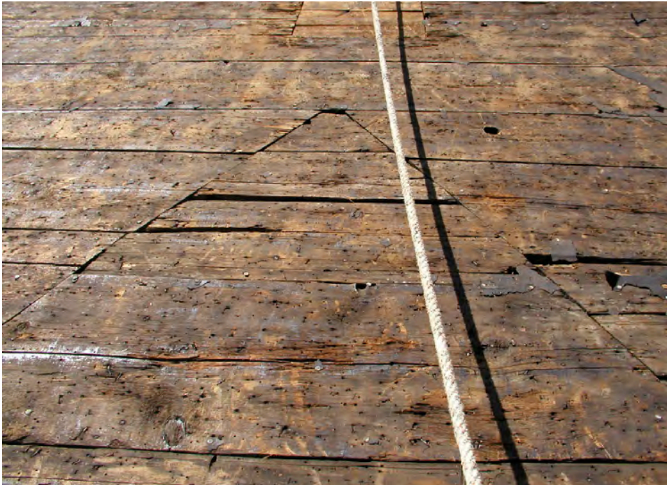
Figure 3. Old Ship Meeting House. East elevation – Patched roof sheathing boards identifying the location of the 1681 roof gable. Rectangular patch above is the former chimney location.
