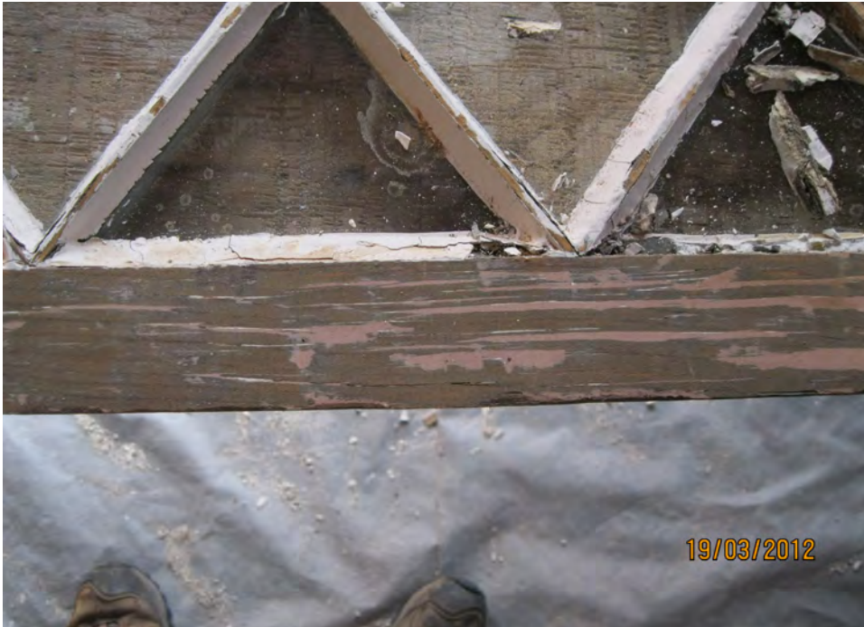
Figure 19. Old Ship Meeting House. 1869 sash – Detail of deteriorated glazing. Photo courtesy of David Webb.
