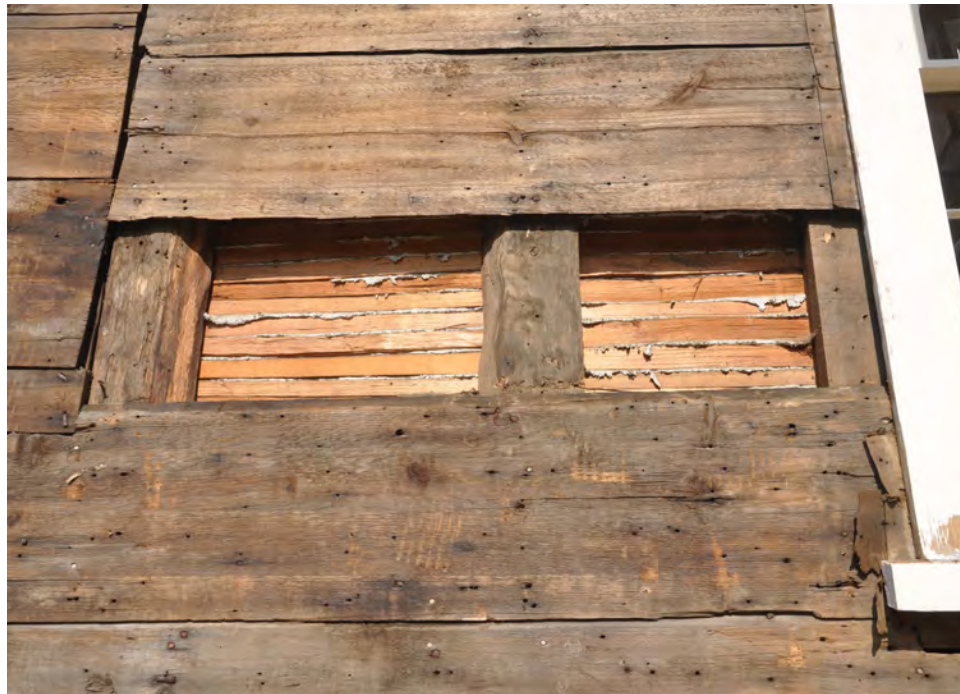
Figure 10. Old Ship Meeting House. East elevation – Detail of casement window (1681) infill. Windows were infilled in 1755.
