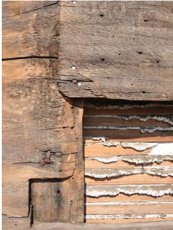
Figure 11. Old Ship Meeting House. East elevation – Detail of casement window infill showing cut-out for window sill.
