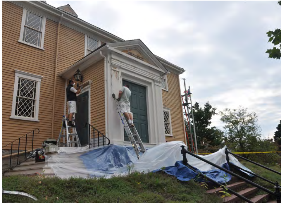
Figure 13. Old Ship Meeting House. Exterior painting – South elevation – Surface preparation.
