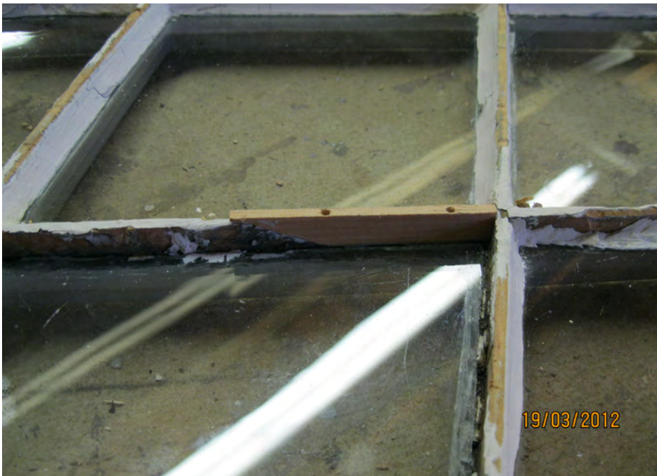
Figure 20. Old Ship Meeting House. Detail of muntin repair. Photo courtesy of David Webb.
