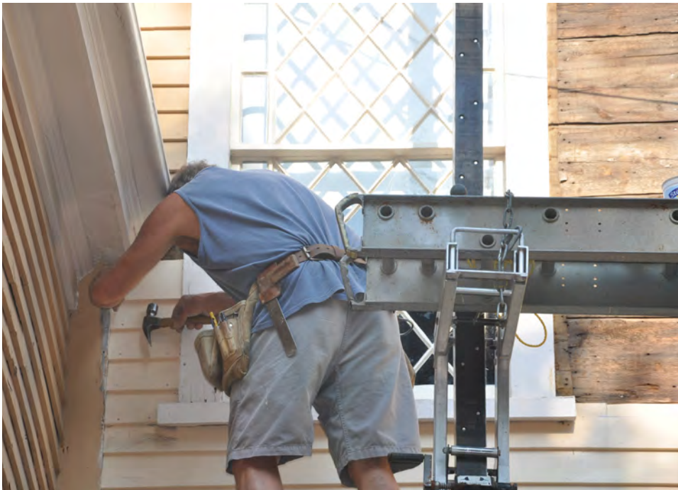
Figure 12. Old Ship Meeting House. East elevation – New clapboards being installed.
