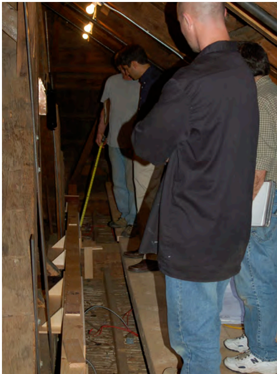
Figure 27. Old Ship Meeting House. Designing the templates for steel fabrication for structural repairs.
