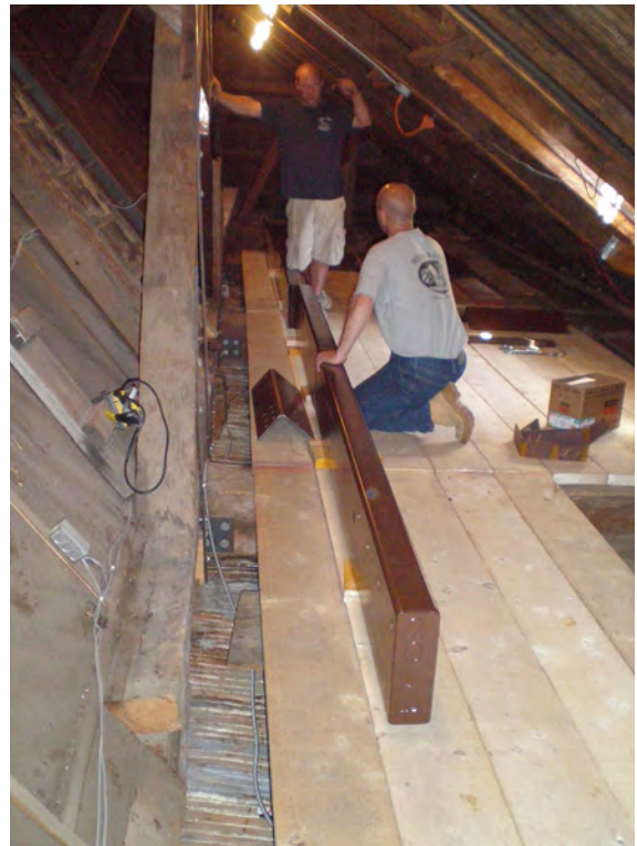
Figure 30. Old Ship Meeting House. Structural steel being prepared for installation.
